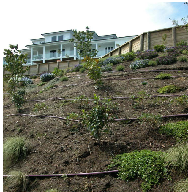
FIG. 2 Drip irrigation pipe prior to bark being laid.
