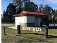
> DARFIELD PUBLIC TOILET
