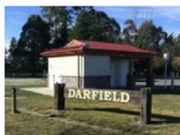
> DARFIELD PUBLIC TOILET
