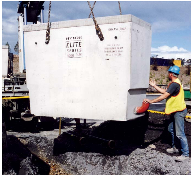
FIG. 1 Grease trap being placed on site
